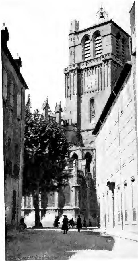
"THE CLOCK-TOWER IS VERY SQUARE AND THICK."—BÉZIERS.
